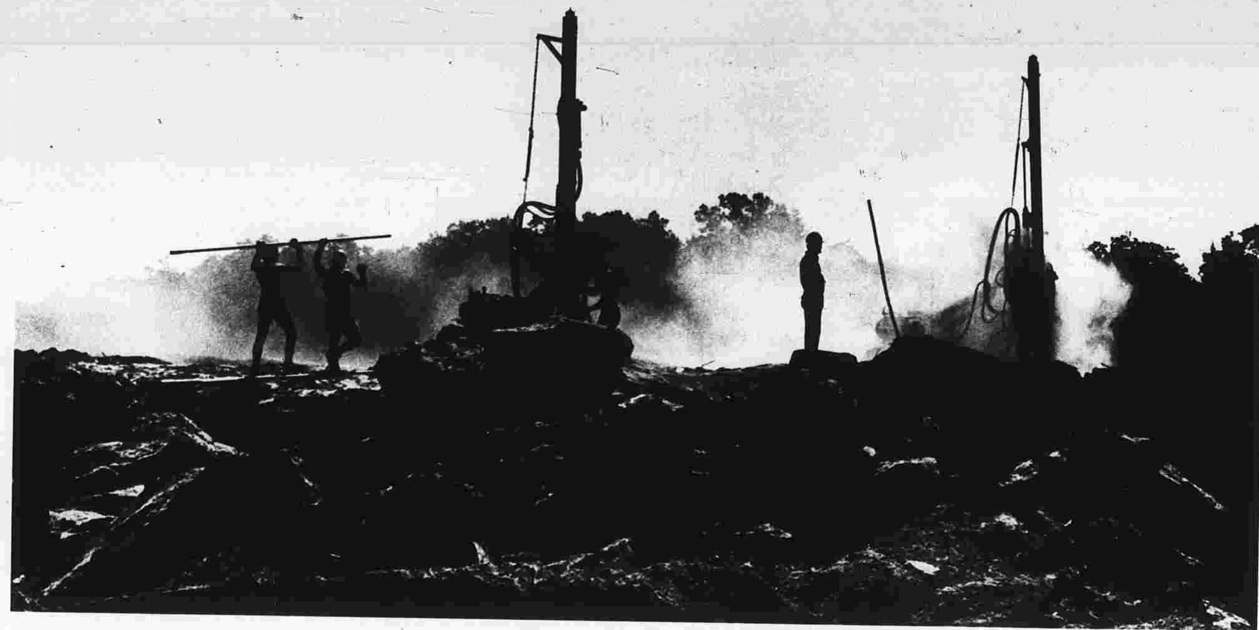
Participating in what resembles an African tribal rite, two shadowy workers carry a spear-like object over their heads as they approach the others drilling through the ledge.
