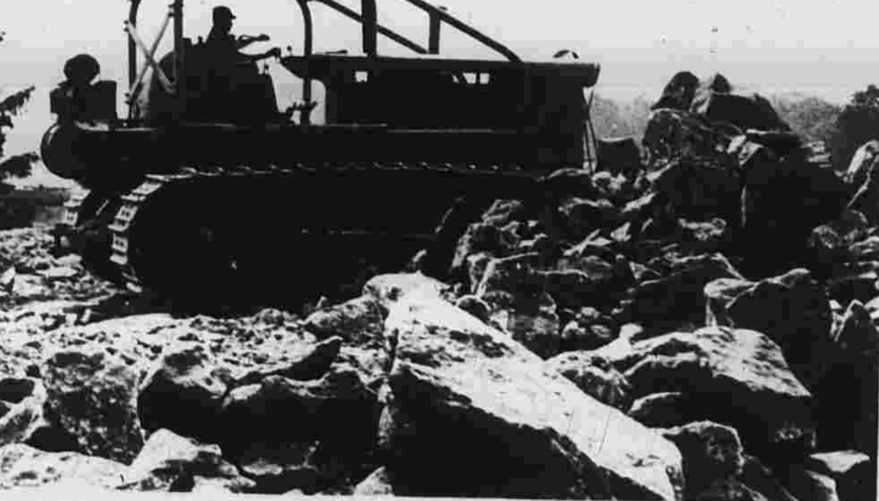
A dozer levels piles of stone dumped by huge Euclids.
